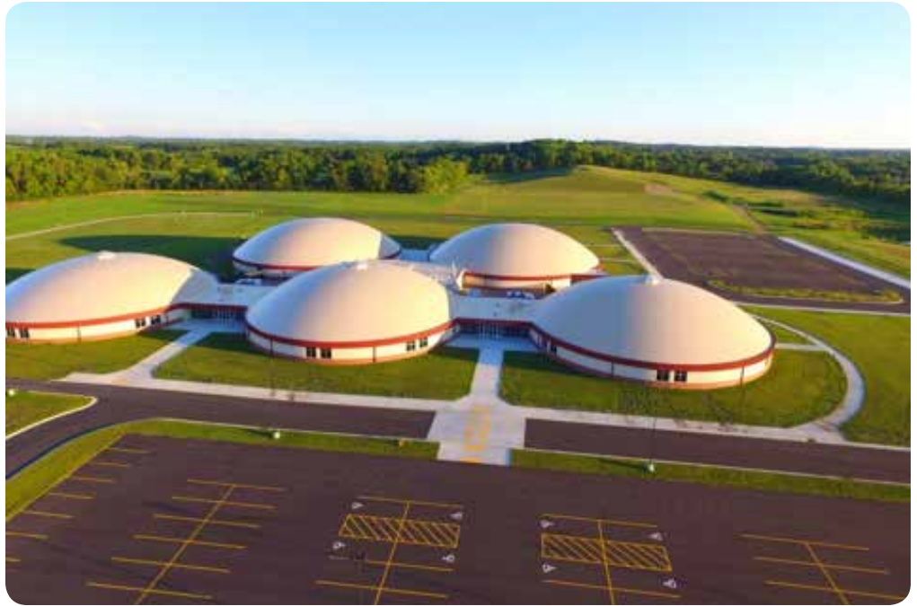
An aerial view of the new facility showing all 5 domes with the interconnecting links. Photo provided courtesy of Mr. Brett Perucco, Tech Integrator and Communications Specialist for Johnson Creek School District.
